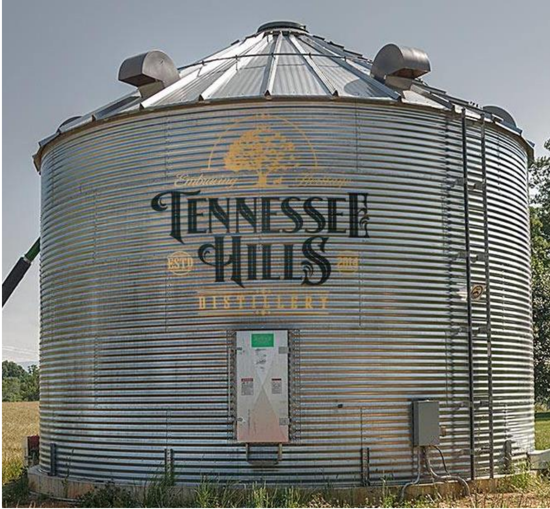
Figure 8. Silo for storing Tennessee Hills Distillery's corn. Tennessee Hills Distillery is bringing a new type of business to a local silo as their demand for corn and corn storage increases in the coming years.
