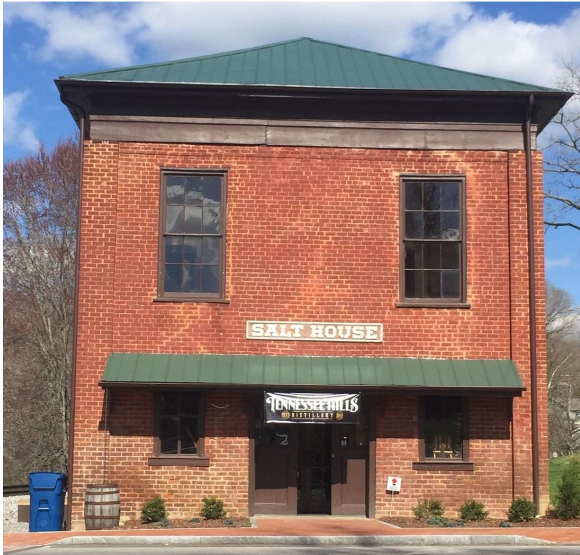
Figure 6. The old salt house where Tennessee Hills Distillery produces and sells commercial moonshine. The 175 year-old building is reflective of the distillery motto, "Embracing Heritage."
